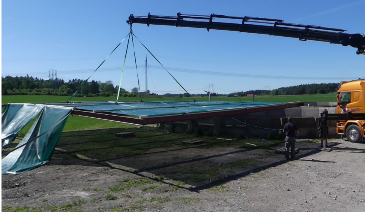
Placing a shadowing construction on a slurry tank
