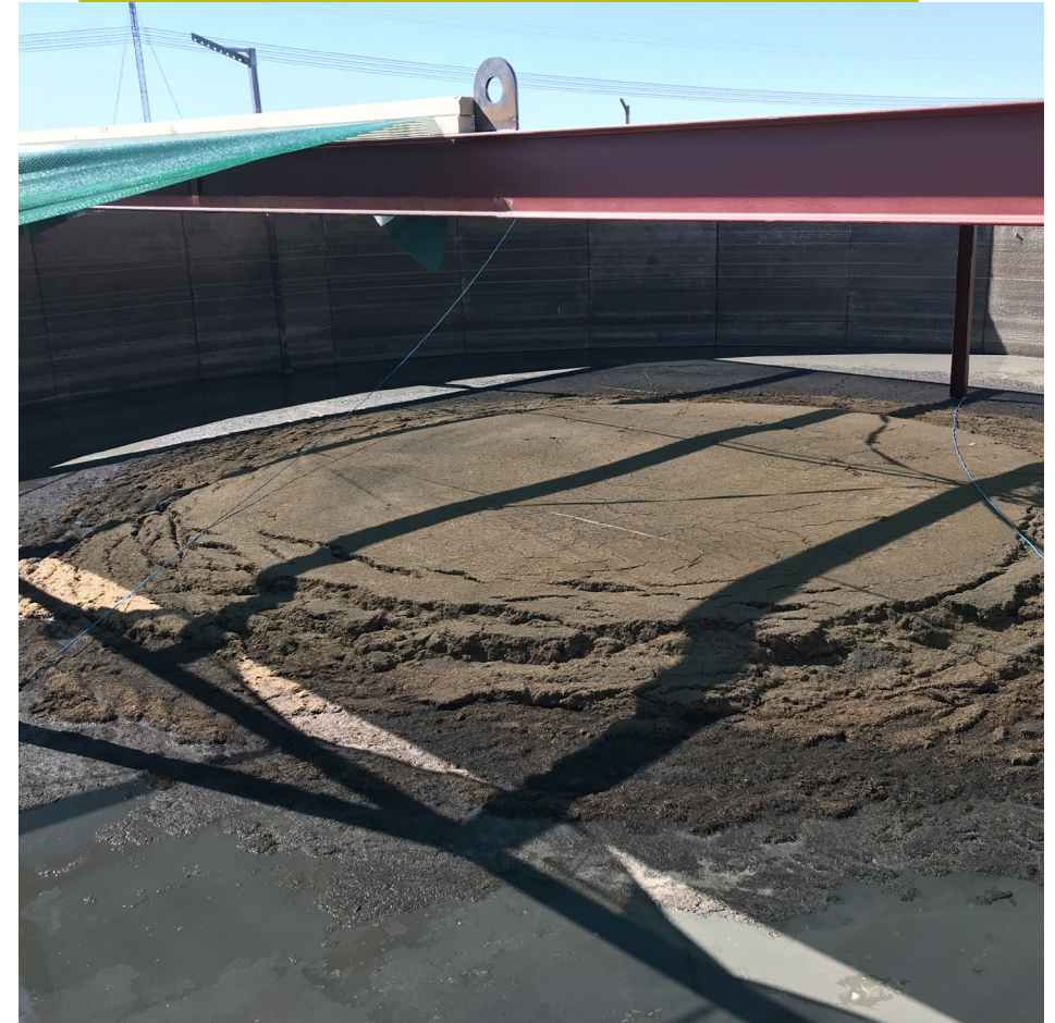
Shadowed slurry surface
